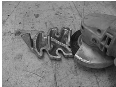
Use metal grinder or other cutter to cut "Marking Studs"
