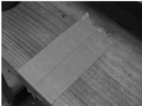
Apply masking tape to surface (sufficiently wide for both studs)
