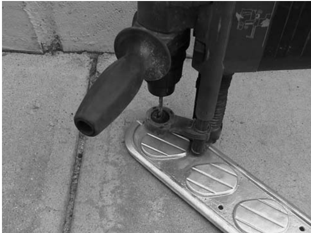
Use part as template to drill first hole
